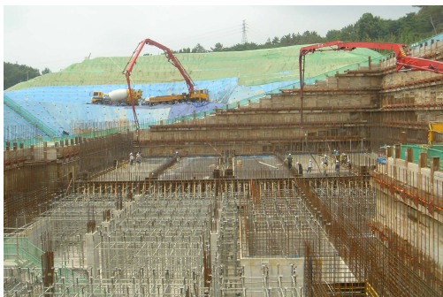
Underground structure concrete works
